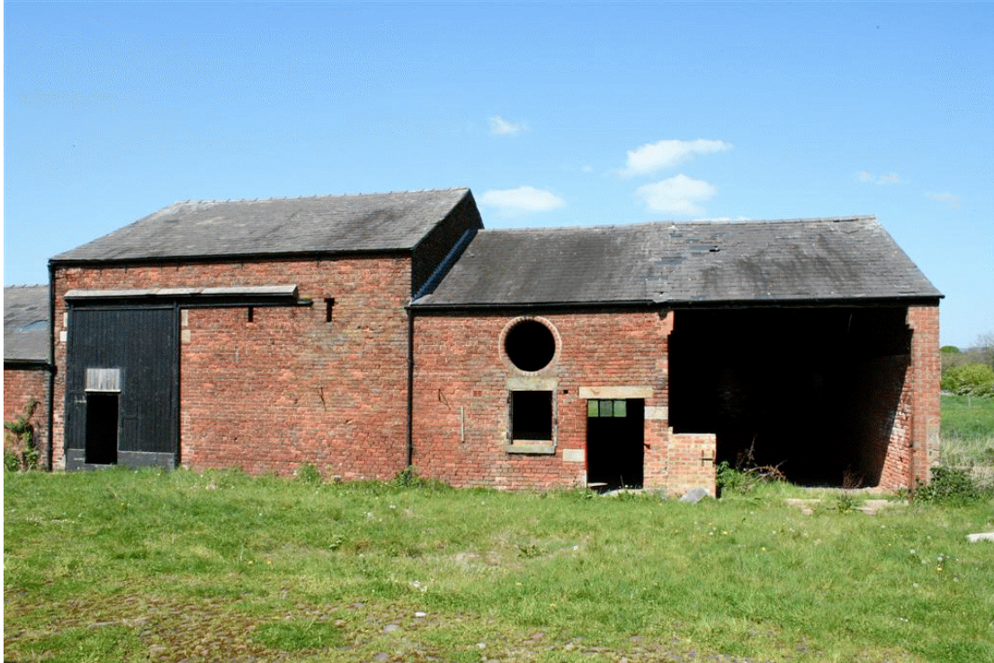
Plate 13: North-facing view of the barns at South Planks, formerly Myerscough Planks (Site 49)
