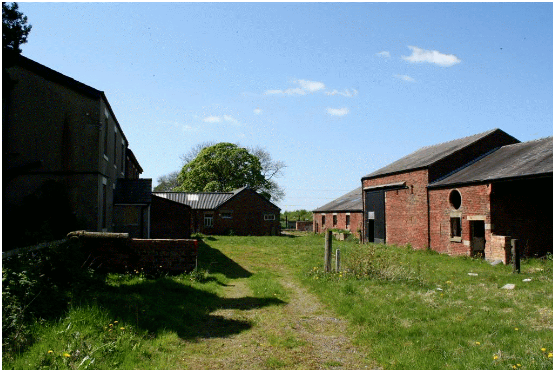
Plate 14: West-facing view of South Planks Farm range, formerly Myerscough Planks (Sites 48-50)
